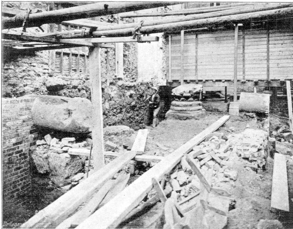
View of Excavations looking East.
